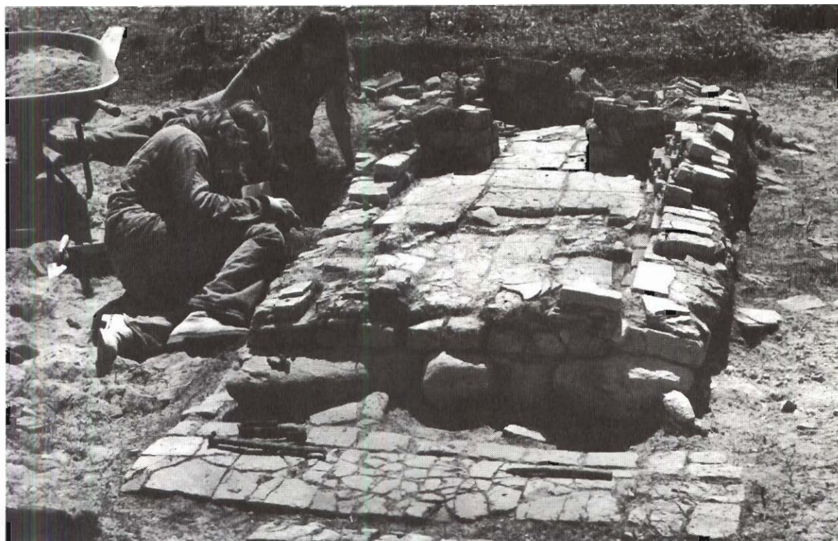
Plate 148 Base of a stove, Charlton Island.
