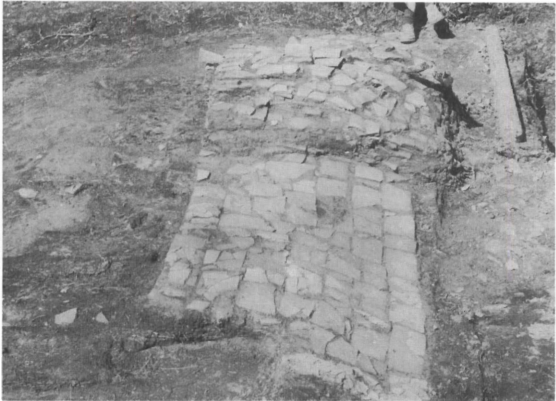
Plate 3 Tile structure, House No. 1, Fort Albany.
